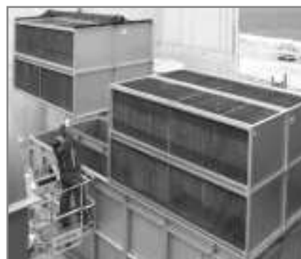
Fig. 13: Plate exchangers installation.
